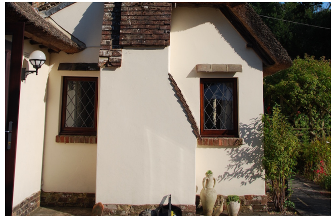
Figure 54 rendered brickwork (Anderson 2018h)
