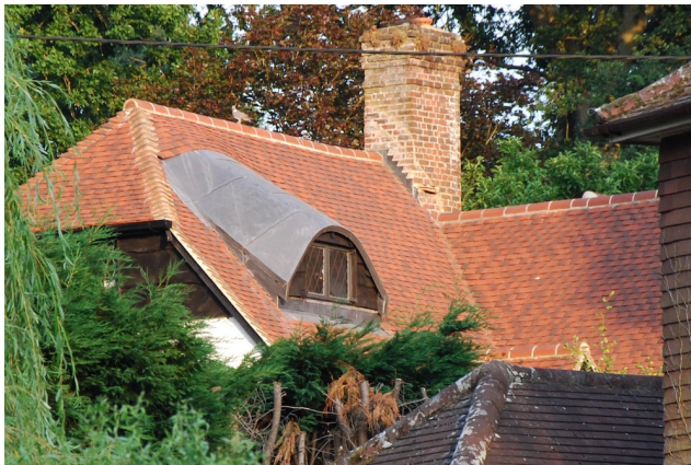
Figure 53 lead covered dormer (Anderson 2018d)
