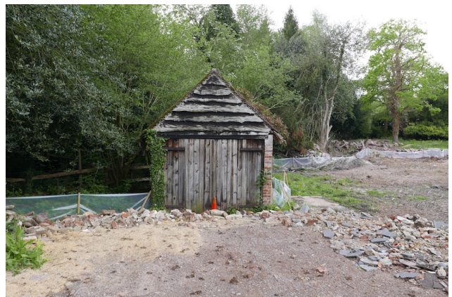
Figure 70 photograph taken prior to demolition (Anderson 2018c)
