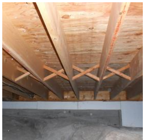
Figure 37 Example of ceiling construction with bracing (Wandel n.d.)
