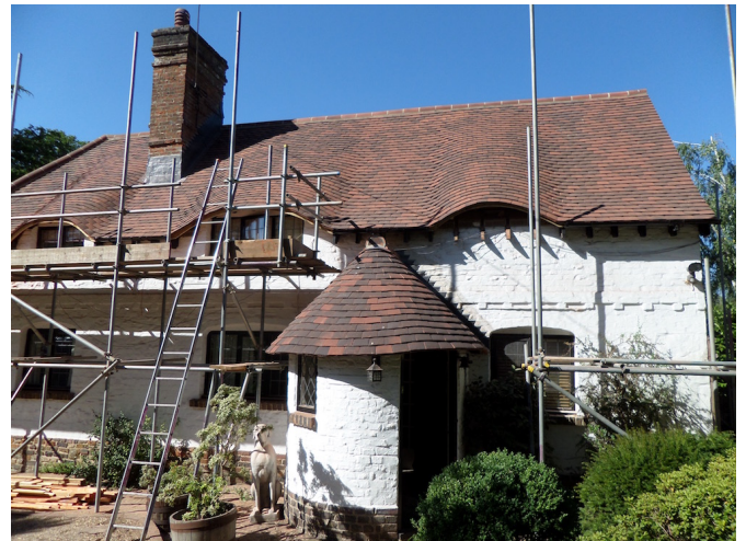
Figure 52 Same cottage as that in figure 51 reroofed (Anderson 2018f)
