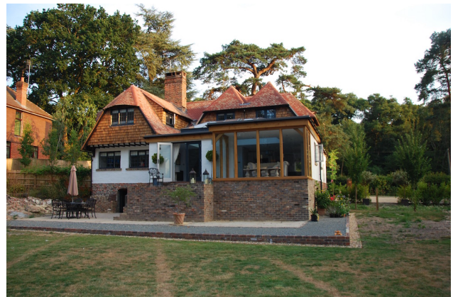
Figure 64 extension confined to the rear (Anderson 2018d)
